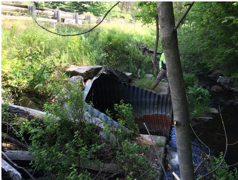
Figure 2. Bridge 51 beneath VT Route 11, looking north.
